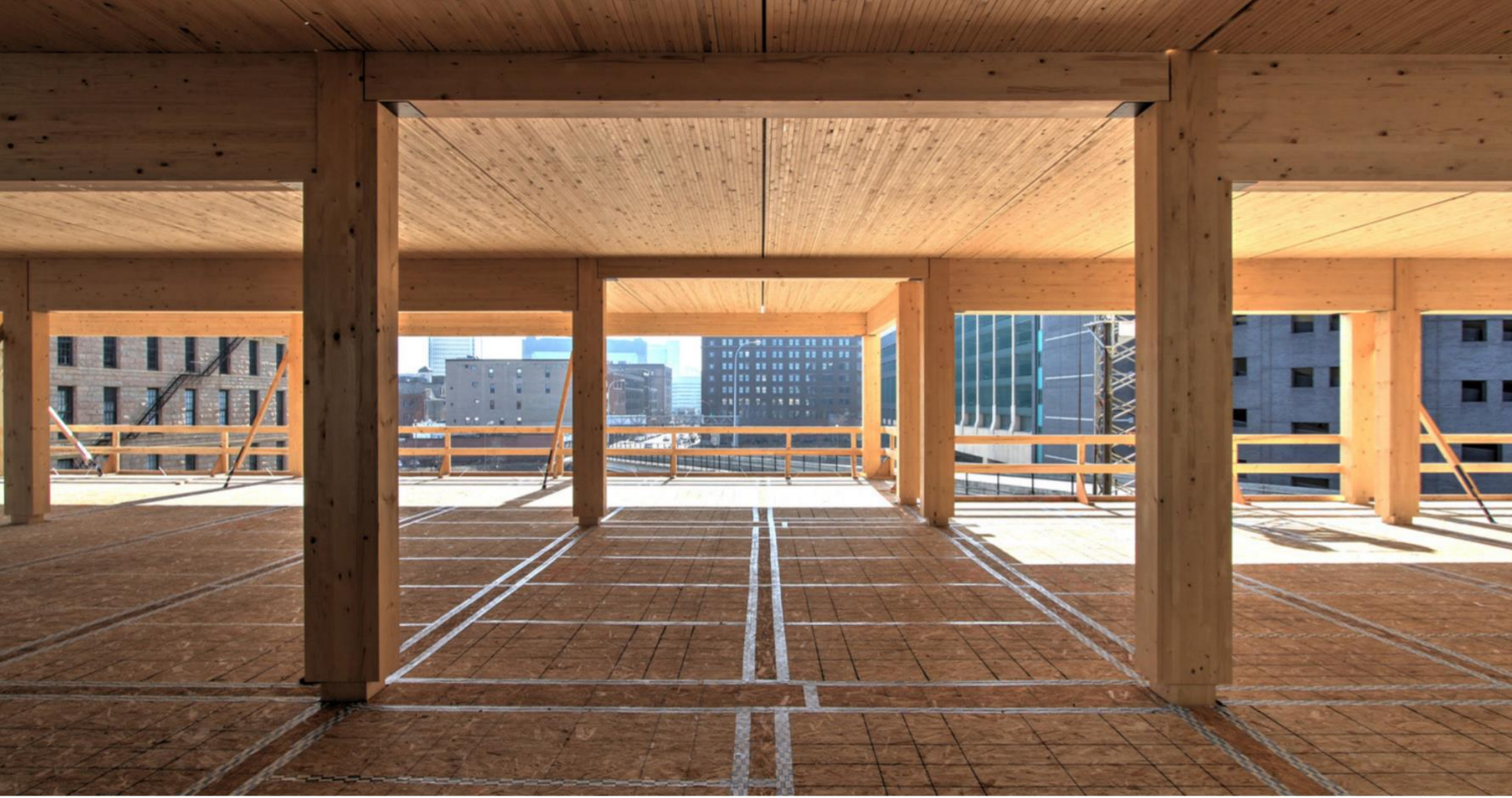
Figure 3.6: Example of exposed wood structure at T3, Minneapolis, MN. Architecture: Michael Green Architecture. (Photo courtesy of Magnusson
