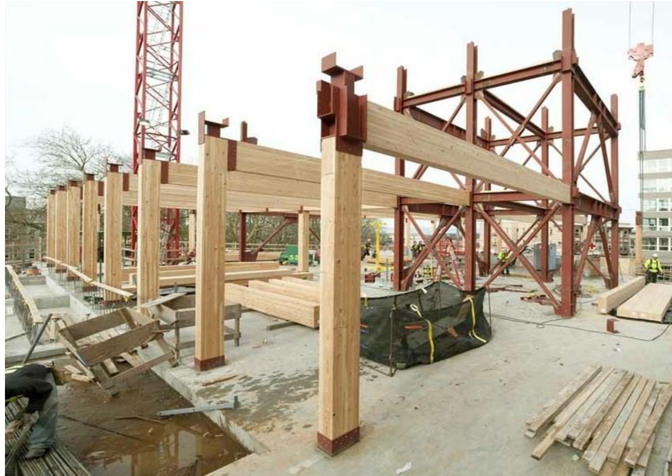
Six story wood framed Bullitt Center, Credit: John Stamets/Bullitt Center
