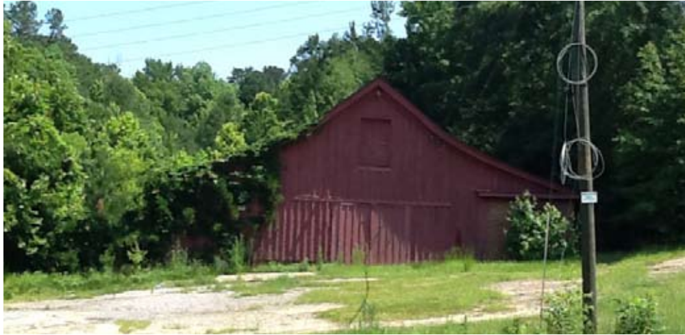
The existing “Red Barn” Property located along Aiken Augusta Highway
